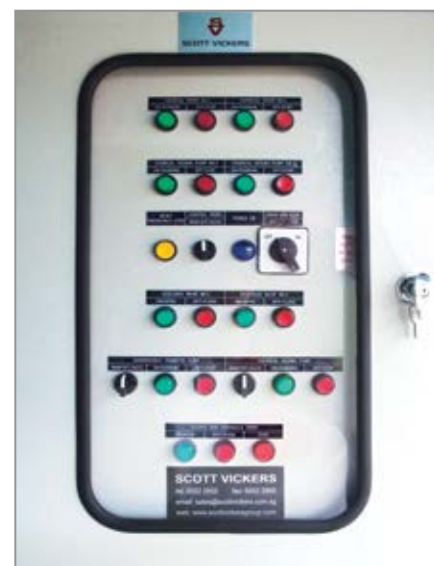
4 The comprehensive but simple single phase Electric Control Panel features individual automatic controls for:- • Chemical Mixers • Chemical Dosing Pumps • Desludge Valves • Sludge Transfer Pump • Sludge Hydraulic Release System
