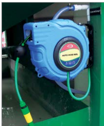
3 Water Hose Reel with automatic hose retraction for cleaning sludge bag, collection tank and lamella blocks
