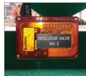
4 Automatic Sludge Discharge Actuator above Liquid Sludge Collection Tank
